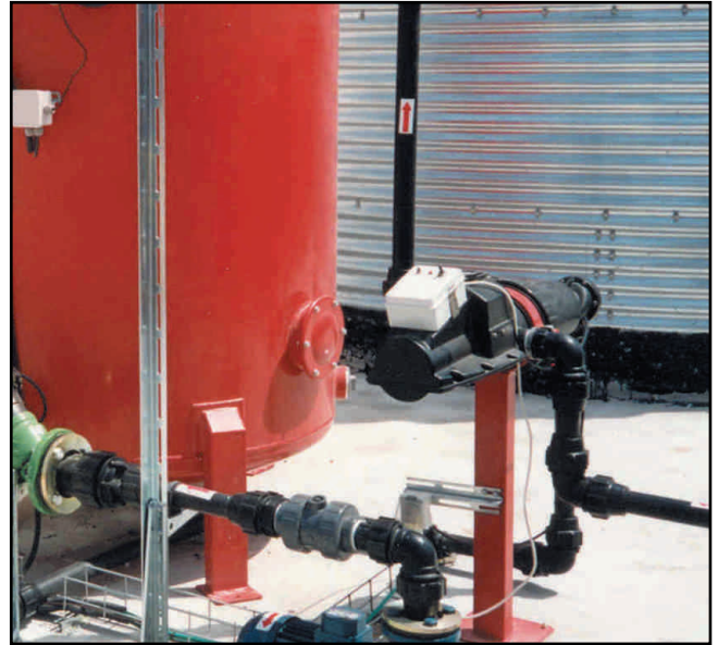
Prefiltration of water treatment plant. Recirculating water at a green house - ISRAEL
