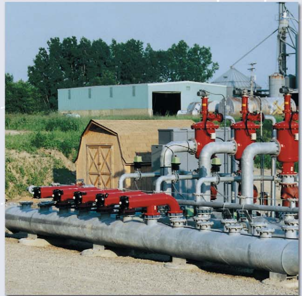
▲ Pre-filtration, Zebra mussel control. Mud-Creek, USA
