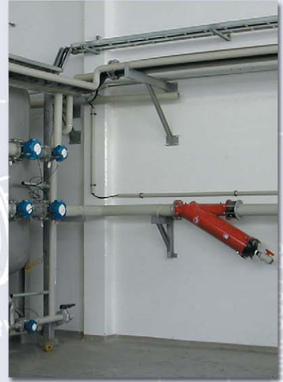
▲ Cooling water filtration. Food manufacturer, Israel
