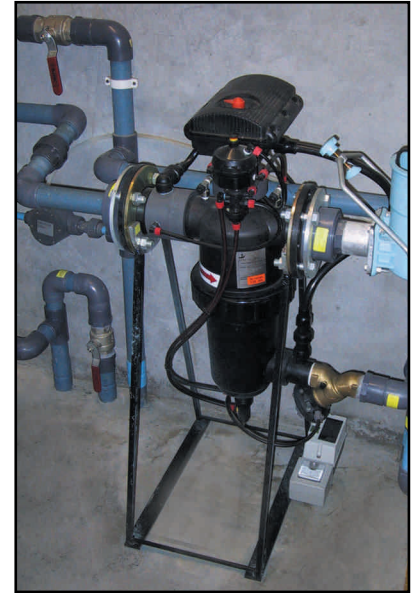
Recirculating water, hot springs SPA - JAPAN
