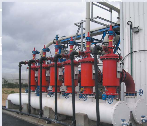
▲ Pre-filtration to RO membranes. 1700m 3 /h, 25µm. Desalination plant, Israel
