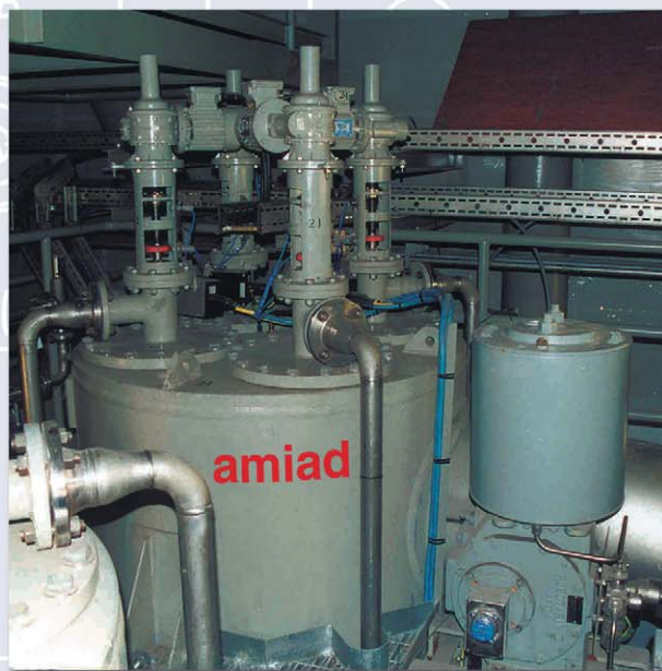
▲ Injection water. 2000m 3 /h, 50µm. North Sea Platform
