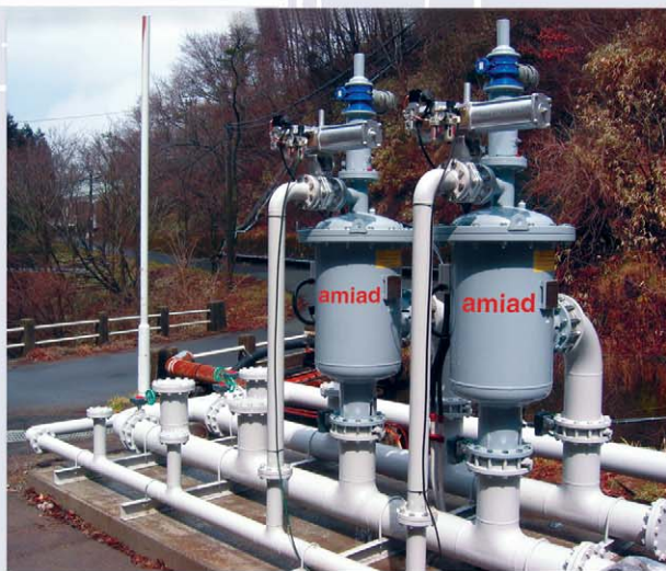
▲ River water for hot spa. 170m 3 /h, 25µm. Japan
