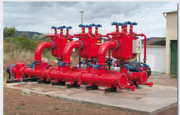
▲ Irrigation water supply. 1800m 3 /h, 50µm. Narbonne, France
