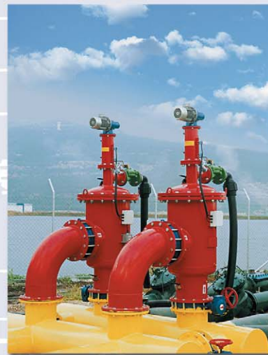
▲ Reservoir water for irrigation. 1000m 3 /h, 100µm. Kfar Hasidim, Israel
