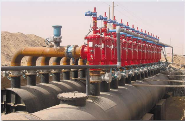
▲ Drip irrigation. 9000 m 3 /h, 130µm. China
