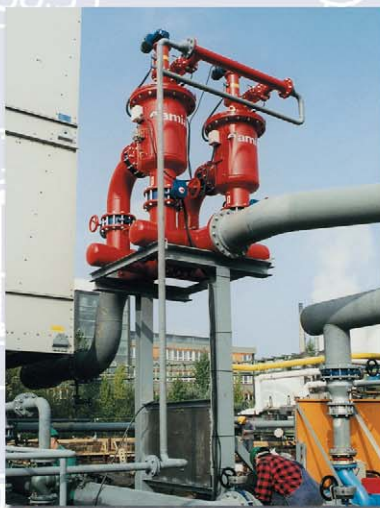
▲ Cooling water in chemical plant. 460m 3 /h, 130µm. Hamburg, Germany
