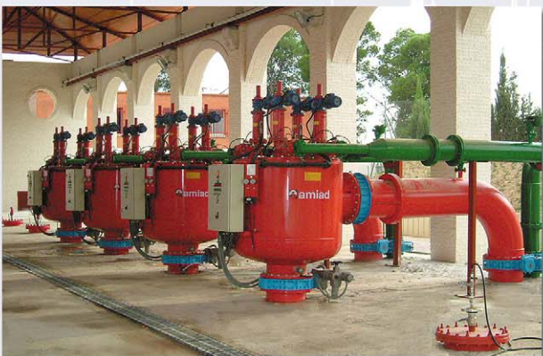
▲ Drip irrigation. 8000m 3 /h, 130µm. Helche Creviente, Spain
