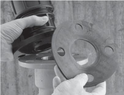
1. Ensure a gasket is used between the flange of the ratio valve and the flange to which it is to be fitted.
