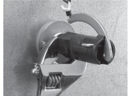
3. Using a pipe wrench or multigrips on the body of the valve screw it into the female thread until tight. Where necessary ensure the female thread is held stationary to avoid it from moving.
