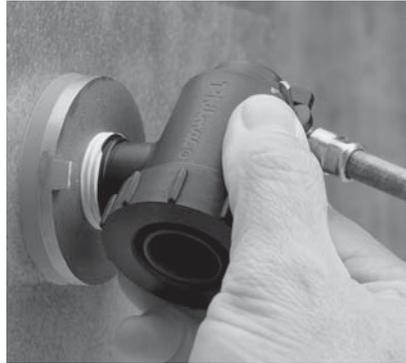
**2.** Screw into female thread by hand until firm\*.
