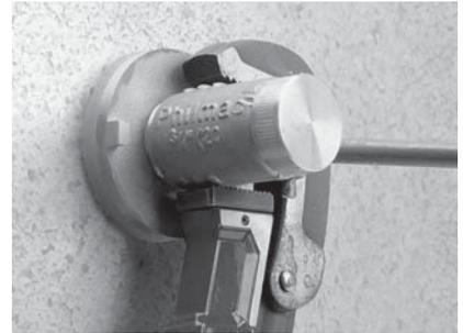
3. Using a pipe wrench or multigrips on the body\*\* of the valve, screw it into the female thread until tight. Where necessary ensure the female thread is held stationary to avoid it from moving.
