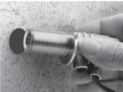
1. Remove the backnut and slide the thread through the appropriate sized hole.
