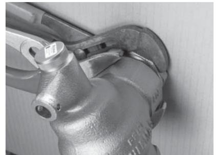
**3.** Using a pipe wrench or multigrips on the hex of the valve, screw it into the female thread until tight. Where necessary ensure the female thread is held stationary to avoid it from moving.
