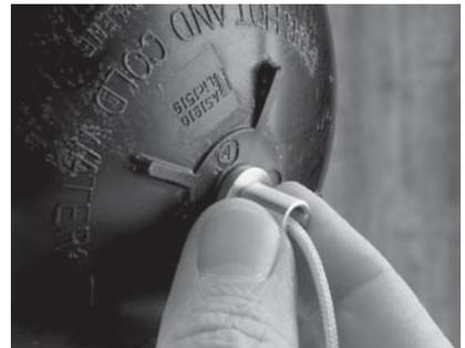
**6.** Re-check and if suitable tighten the female end with a pair of pliers or multigrips so the flange is hard up against the float (ball).
