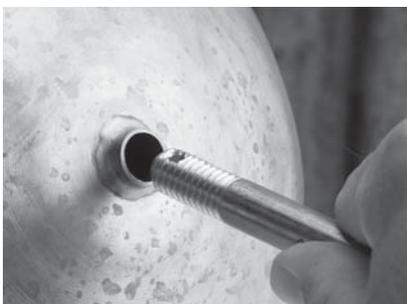
**4.** Thread the lever arm through a 10" (255 mm) copper float (ball) and tighten.
