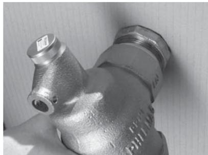
**2.** Screw into female thread by hand until firm.
