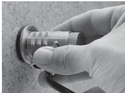
2. Where using the stem sleeve to fit the valve into  $\frac{3}{4}$ " holes, ensure it is properly located on the valve side of the installation to prevent the valve moving.
