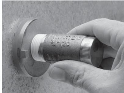
2. Screw the valve into the female thread by hand until firm\*.
