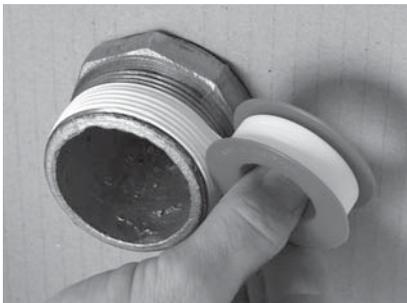
**1.** Apply PTFE tape or approved sealant to the inlet thread ensuring sufficient is applied to ensure a watertight seal.
