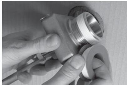
**5.** Apply PTFE thread tape or approved sealant to the inlet thread on the valve and screw it into the tank outlet. Tighten the body using a pair of multigrips or spanner.
