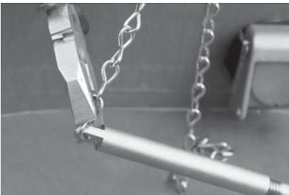
**4.** Cut the stainless steel jack chain to the required length and fit it to both the arm extension and the float adaptor. It may be better to leave the chain slightly longer as it can subsequently be cut to the exact length after a trial fitting. If necessary adjust the length of the jack chain to ensure the trough has the required level of water.
