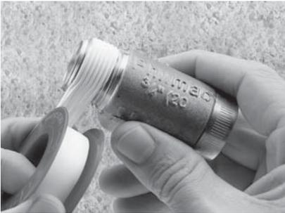
1. Apply PTFE tape or approved sealant to the thread ensuring a sufficient amount is applied to guarantee a watertight seal.
