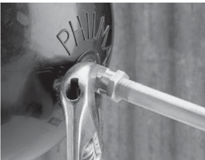
4. Screw the male end of the adaptor into the 8" (200mm) float (ball) and tighten fully using a spanner.
