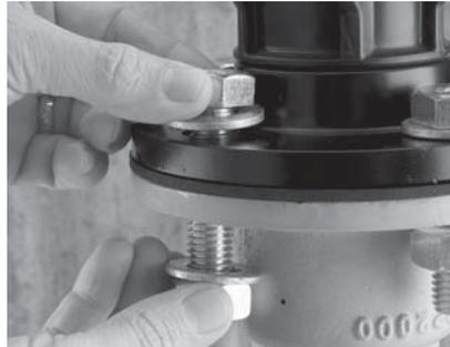
2. Fit the correct size and length bolts to each hole in the flange and hand tighten them.
