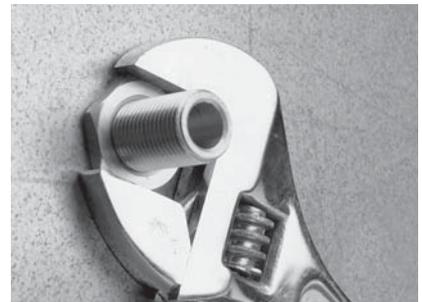
3. Refit the backnut and tighten with a spanner. The valve body\*\* can be held in place with a spanner, multi-grips or equivalent.
