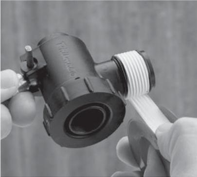
**1.** Apply PTFE tape or approved sealant to the thread ensuring sufficient is applied to ensure a watertight seal.
