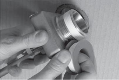
**1.** Apply PTFE thread tape or approved sealant to the inlet thread and screw the valve into the tank outlet.
