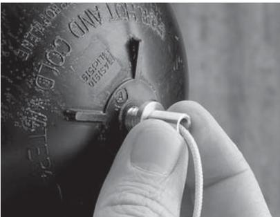
**4.** Screw the male end into the appropriate sized float (ball) and hand tighten to the flange.
