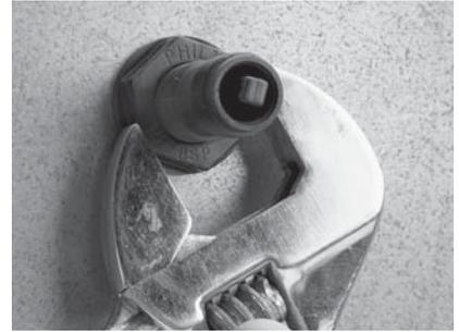
3. Screw the back nut onto the thread and tighten.
