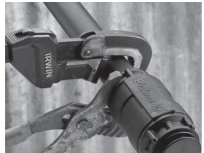
**3.** Using a pipe wrench or multigrips on the end caps only, further screw the air relief valve into the male thread until tight. Where necessary ensure the male thread is held stationary to avoid it from moving.
