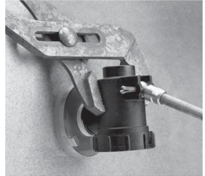
**3.** Using a pipe wrench or multigrips on the body\*\* of the valve screw it into the female thread until tight. Where necessary ensure the female thread is held stationary to avoid it from moving.
